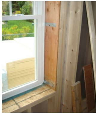
PHOTO 3 Strap Window Attachment. Similar to window installation in masonry openings lined with window bucks. Unlike masonry openings the window flanges are retained for water control. FIGURE 7 Structural Box. Note that with the structural box the water control layer is wrapped into the box opening and the material is typically flashing tape.
