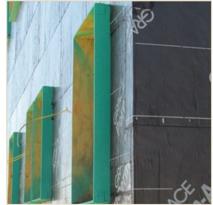
PHOTO 2 Structural Box. Typically plywood or OSB protruding past the exterior face of the framing, extending the thickness of the continuous insulation. How thick can you go with the continuous insulation with the structural box? Typically 4 to 6 in.
