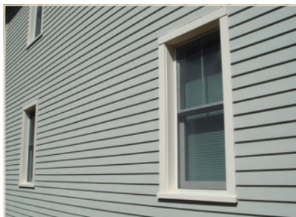
PHOTO 1 Beautiful “Innies.” The trim is returned to the flange or face of the inset window. The flashing at the top of the window opening at the horizontal strip of head trim just covers the top of the trim itself—it only protects the top of the trim—it does not have to extend to the back of the continuous insulation and connect to the face of the structural sheathing/water control and air control layer.
