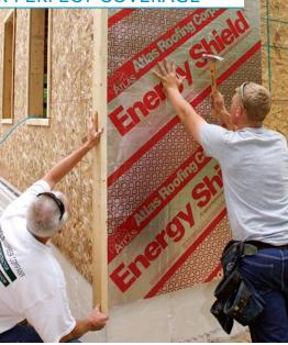
Marking the panels in place is easier than measuring. Around rough openings, it's just as quick and more accurate to lift the panels into place to mark them rather than take measurements. Mark the panel for the horizontal cuts, and measure the distance from the furring strip to the closest panel for the vertical cut. Use a T-square to draw cutlines, and cut through the panel in one pass with a heavy-duty snapblade knife (www.tajima tool.com).
