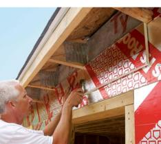
materials I typically use. When I decided to include rigidfoam insulation in wall assemblies, I had to consider how it would affect the entire wall system. For instance, the foilfaced polyisocyanurate used here is a vapor barrier, so I eliminated the interior vapor barrier of the original design.
