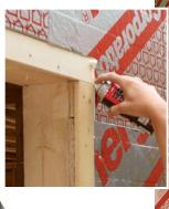
back and fasten the panels every 12 in. on center around the edges and 16 in. on center in the field. Manufacturers recommend fasteners with at least a <sup>3</sup>/<sub>8</sub>-in. head, so I use aluminum roofing nails. Cap nailers also work well.
