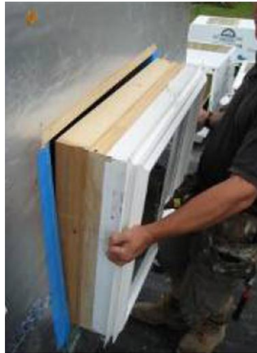
Image 2.4: Extension Jambs attached directly to a window
