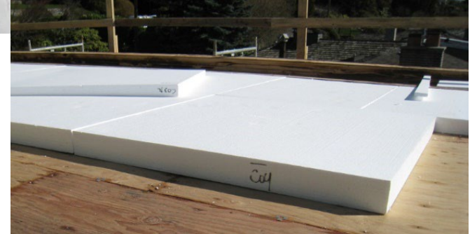
Above deck roof insulation installation
