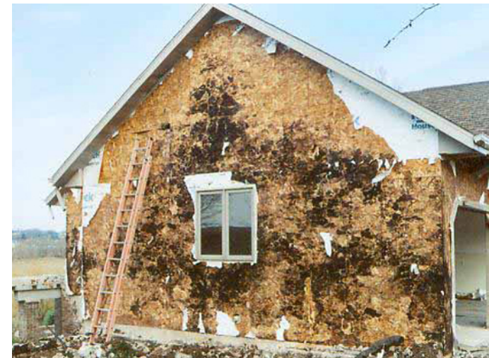
Inward Moisture Movement Due to Solar Radiation
