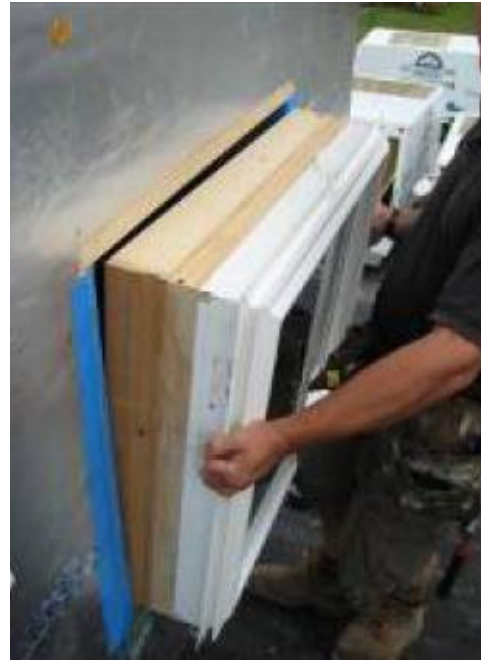
Image 2.4: Extension Jamb attached directly to a window
