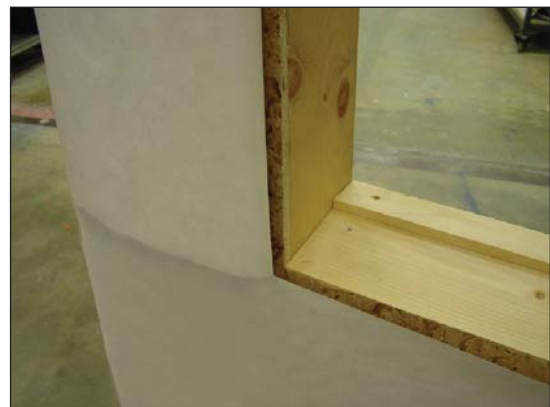
Figure 5. Sloped sill and back dam
