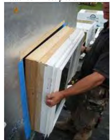
Figure 14. Extension Jamb Attached Directly to a Window
