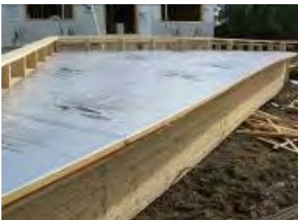
Figure 16. Rigid Foam Applied to Gable End on the Ground then Lifted into Place with a Crane
