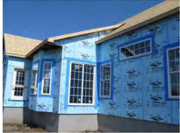
Figure 9. Home in New York Covered with 2” of Rigid Foam
