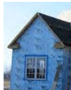
Figure 17. Rigid Foam Continued over Gable End
