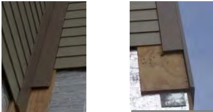
Figure 13. Sliding Plywood at Inside and Outside Corners
