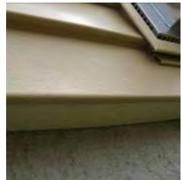
Figure 15. Capped Foam Edge at the Bottom of a Wall with Metal Flashing
