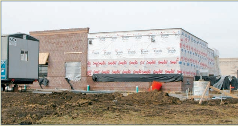
Figure 2. Commercial construction project using polymeric WRB behind brick veneer.
