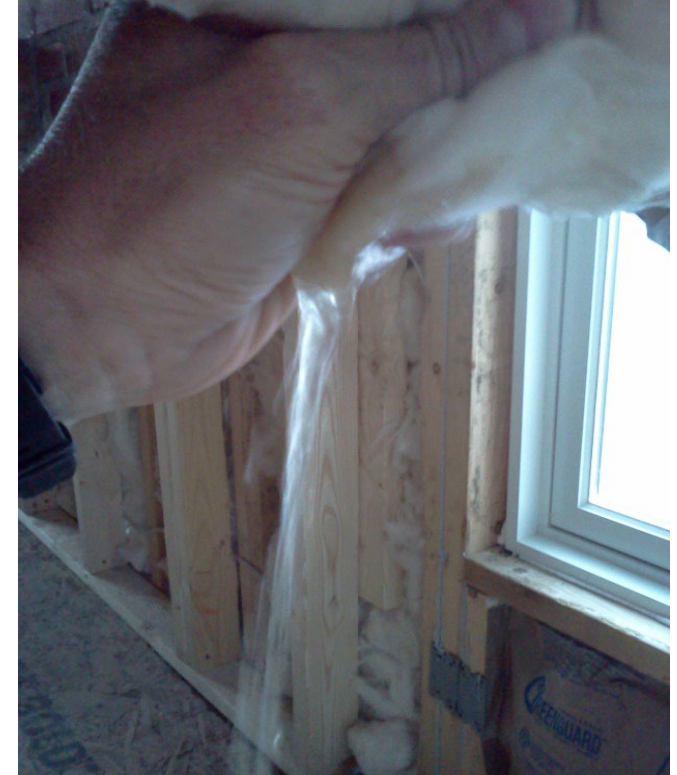
Storm water expelled from FG batt insulation installed prior to completion of the WRB and flashing
