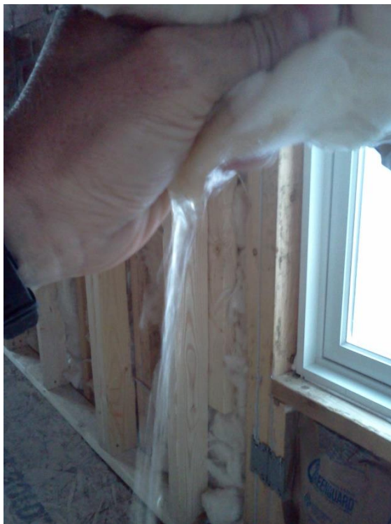
Figure 8. Initial Construction Moisture (Intruded Rain Water) Being Expelled from Fiberglass Batt Cavity Insulation Due to Poor Construction Sequencing (e.g., cavity insulation installed prior to dry-in of the exterior wall with, at a minimum, a complete installation of the exterior water resistive barrier and flashing).
