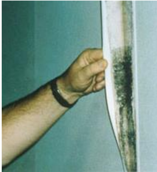
Figure 5: Mold Behind Vinyl Wall Paper – Vapor Retarder on the Wrong Side in Warm/Humid Climate (Source: https://www.epa.gov/mold/brief-guide-mold-moisture-and-your-home )
