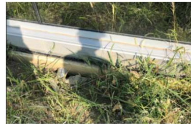
Photo by Shaunna Mozingo (commonly uninsulated slab edge or unprotected if placed on exterior side)
