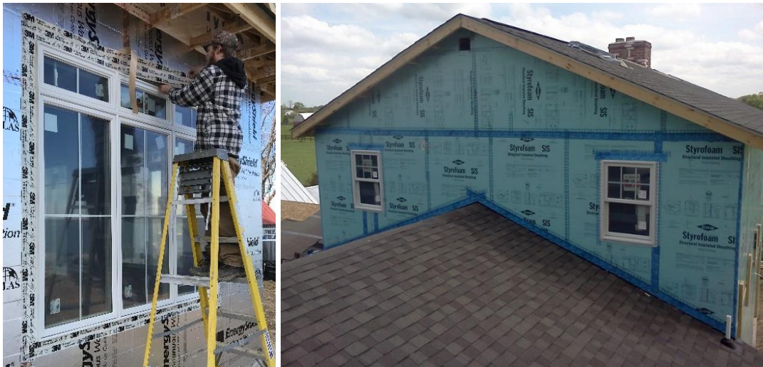
Figure 3. Adhered flashing and joint tapes used for FPIS WRB systems and window flashing for houses completed in 2014 and 2019.
