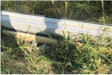
Photo by Shaunna Mozingo (commonly uninsulated slab edge or unprotected if placed on exterior side)
