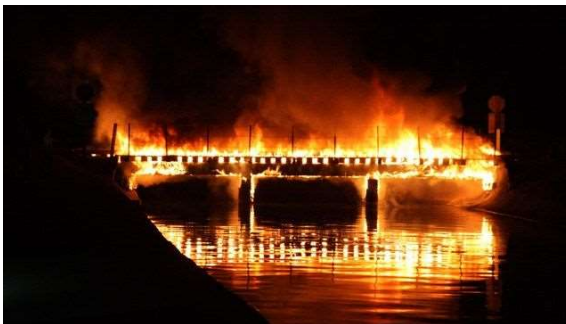
Burning bridge releasing the embodied (stored) energy. Source: Steve Dadds; as published in azfamily.com by 3TV/CBS 5, posted Aug. 17, 2015.
