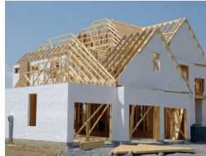
House wraps = 5 to 50 perm (depending on type)
