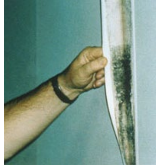
Low perm interior finish on interior (warm-in-winter) side of wall in hot/humid climate – perfect for culturing mold colonies!
