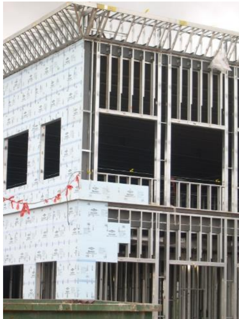
Thermal bridging in steel framed wall with cavity insulation and foam plastic insulating sheathing (FPIS) continuous insulation (ci).
